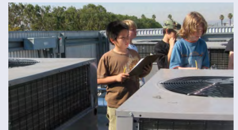
Students survey the school's HVAC units.
